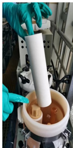
Figure 9. Filter check after 3 months continuous operation
