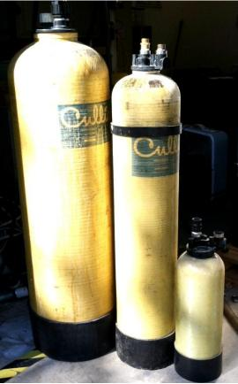
Photo 1 Fiberglass absorptive media tanks (2.5ft<sup>3</sup>, 1.5ft<sup>3</sup>, 1/4ft<sup>3</sup> shown)
