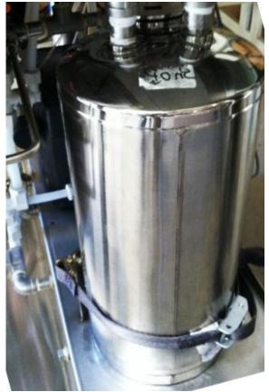
Photo 2 Stainless absorptive media tank (½ ft<sup>3</sup> shown)
