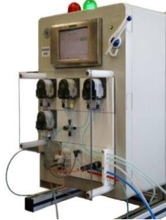
Figure 11 Analysis unit for copper and redox system
